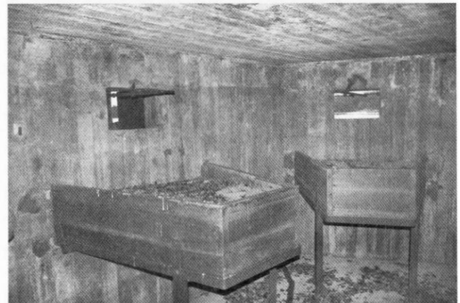
Raised sand boxes for heavy machine gun tripods in an isolated pillbox on Arholma island.
